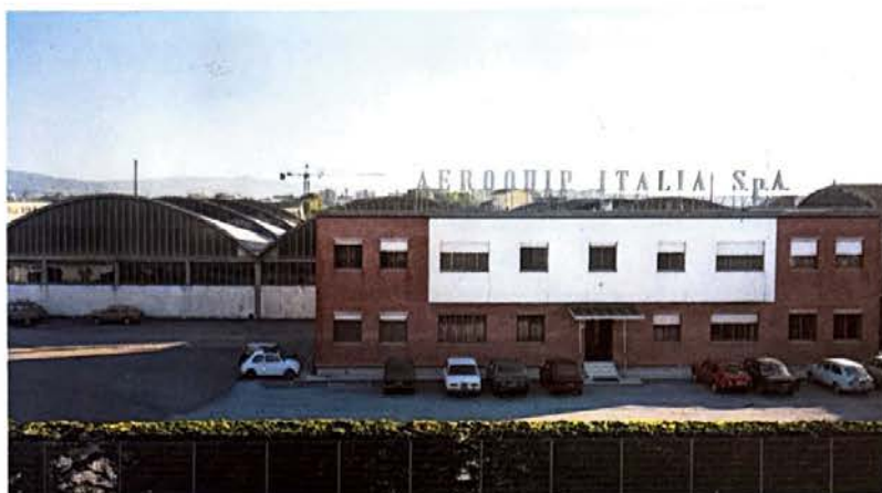
Pictured left are the offices and plant of Aeroquip Italia S.p.A. which are located at Livorno, near Pisa on the Mediterranean coast.
